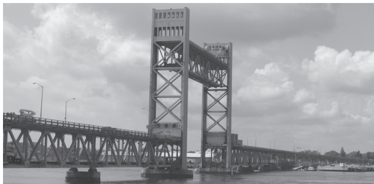
In 2009, Yates Electric completed the project for the NH Dept. of Transportation and the Interstate Bridge Authority. The project involved a complete upgrade of the Bridge's lift and control systems.
