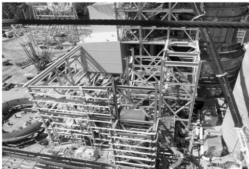
Fluidized gas desulfurization building in progress.
