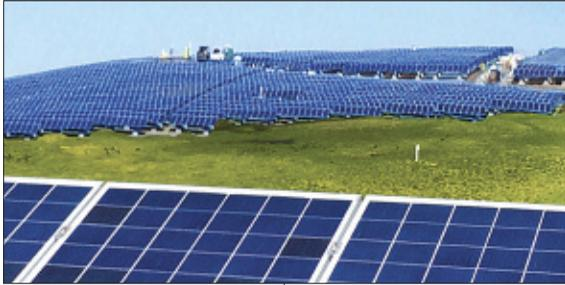
solar energy facilities totaling over 12MW of power on Cape Cod for the Cape and Vineyard Electrical Cooperative, Inc. The solar facilities were constructed on capped landfills in the towns of Barnstable, Chatham, Dennis, and Brewster.
