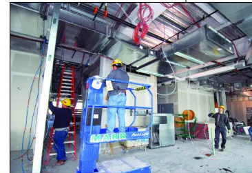
Electrician guides cable over mechanical equipment before cable is supported
