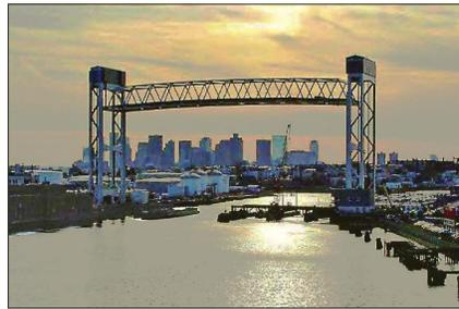
220 feet above the ground, which house the majority of the electrical equipment. Once the old bridge was removed, the job was separated by the waterway, requiring separate crews and equipment in both towers.
