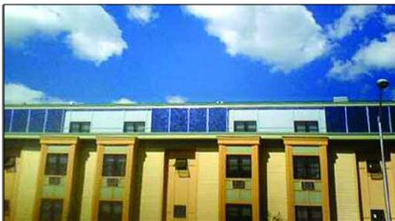
connected right up to the metal drip edge of the building. This solar system design and installation ideally shows the ability to meet unique project demands and concurrently build a solar system with limited roof space. A vertical PV system was added to the front of the building, adding to the system's electrical capacity and further demonstrating the commitment to solar. ■
