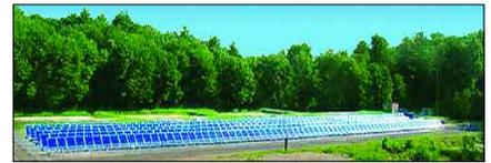
system. The PV modules are supported by ground-mount structures made of formed aluminum channel with an integral ballast system. The structure's design lends itself to quick assembly and rapid alignment and installation of the PV modules at a fixed orientation and tilt angle.
